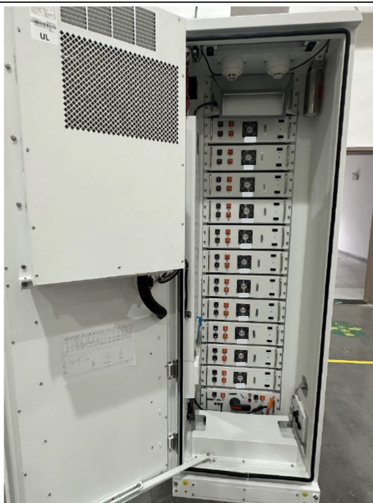
Figure 5. Internal view of battery unit (L3 HVR-60)
